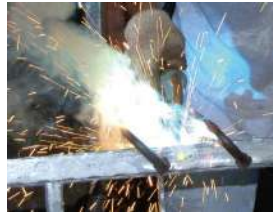
溶接・組立て
